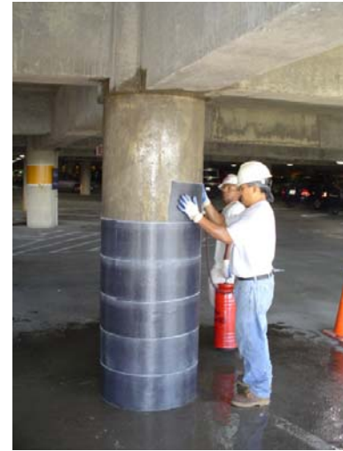
Figure 5: Column Bolstering. Courtesy: RGA
