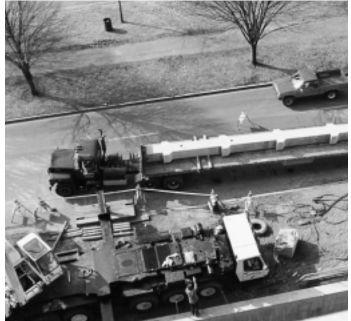
MEGA-SPAN™ Columns are delivered as single units up to 75' long.
