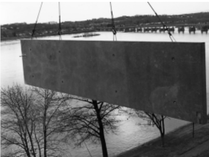
Shear Wall sections are installed as monolithic units of up to 13'-8" x 45'.
