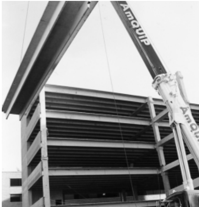
MEGA TEES™ are placed into pockets in Exterior Spandrels.
