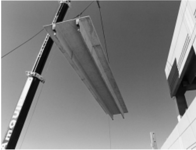
Crane lifting MEGA TEE™ into position
