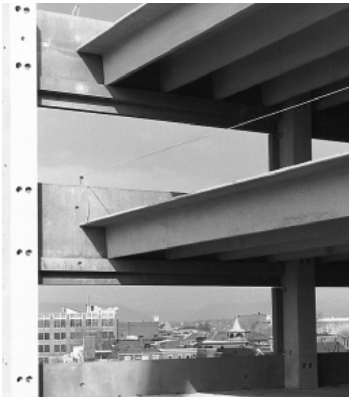
MEGA TEE™ bearing on Spandrel
