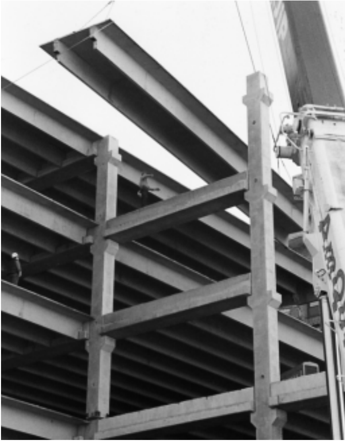
MEGA-SPAN™ components are easy to erect. Columns and Girders are installed first.
